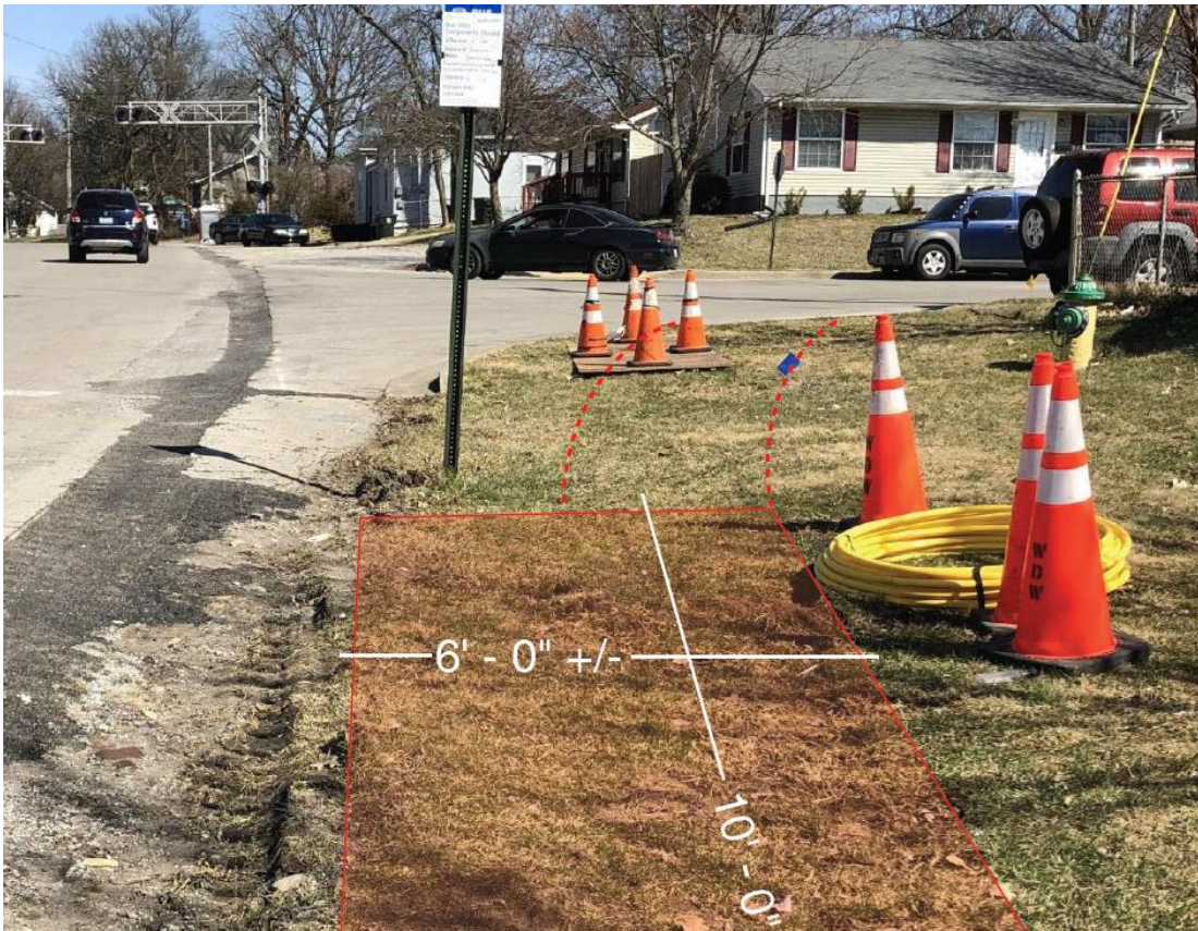
Figure 5-4. Shropshire at Shelby Outbound Stop Boarding Pad Construction
